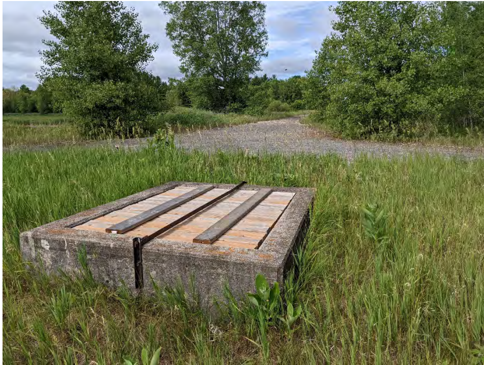
Image 15: Sewer utilities, looking west
