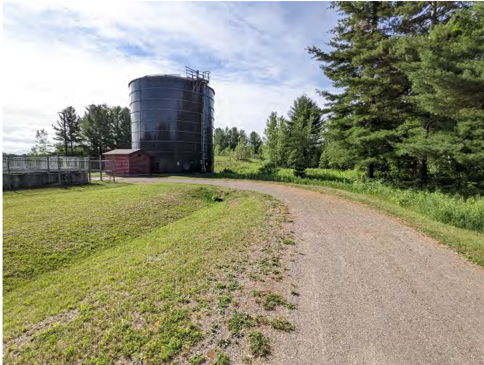
Image 3: Disturbed. Heavily modified landscape, drainage ditches and above/below ground utilities/facilities, looking south-southeast
