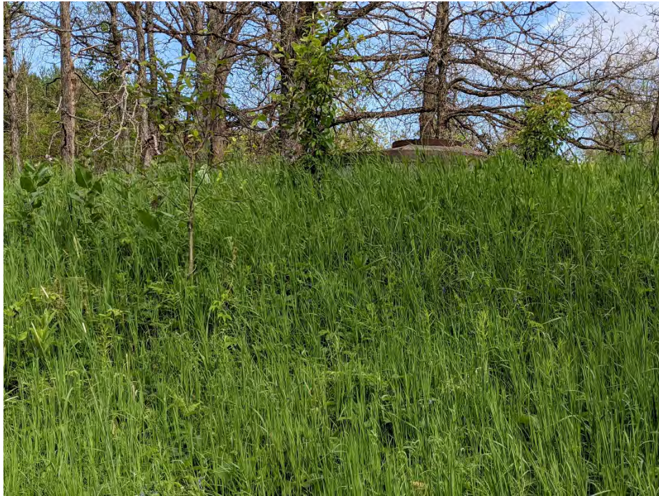
Image 19: Disturbed. Exposed manhole cover atop earthen berm, looking north
