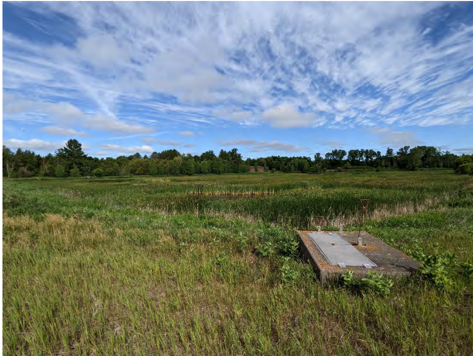
Image 9: East settling pond and sewer utilities, looking northeast
