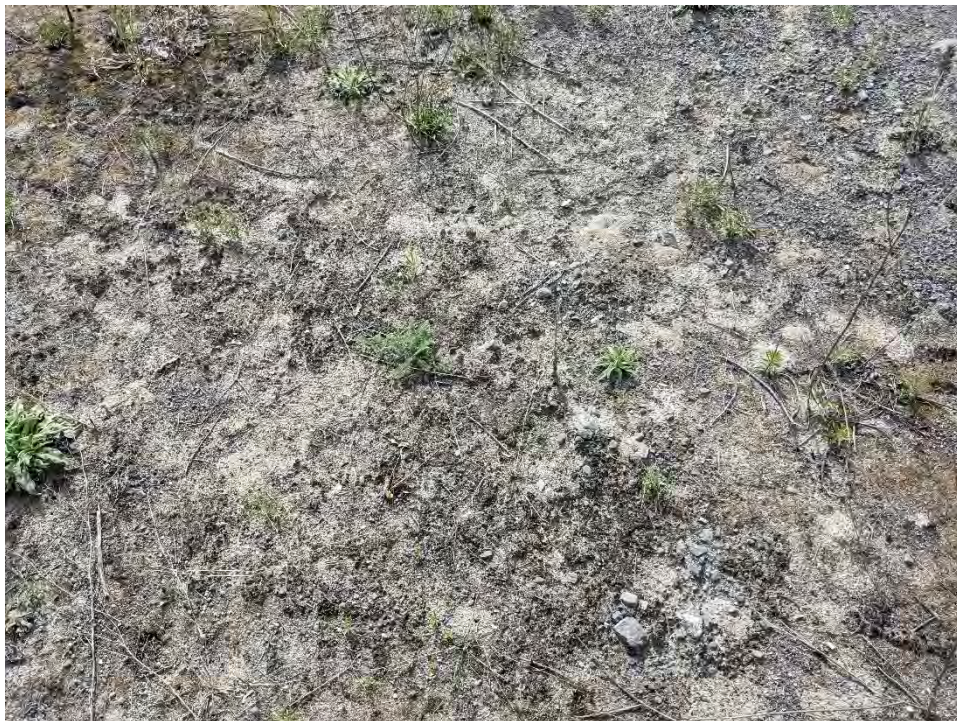
Image 12: Disturbed surface soil conditions surrounding the settling ponds, looking down
