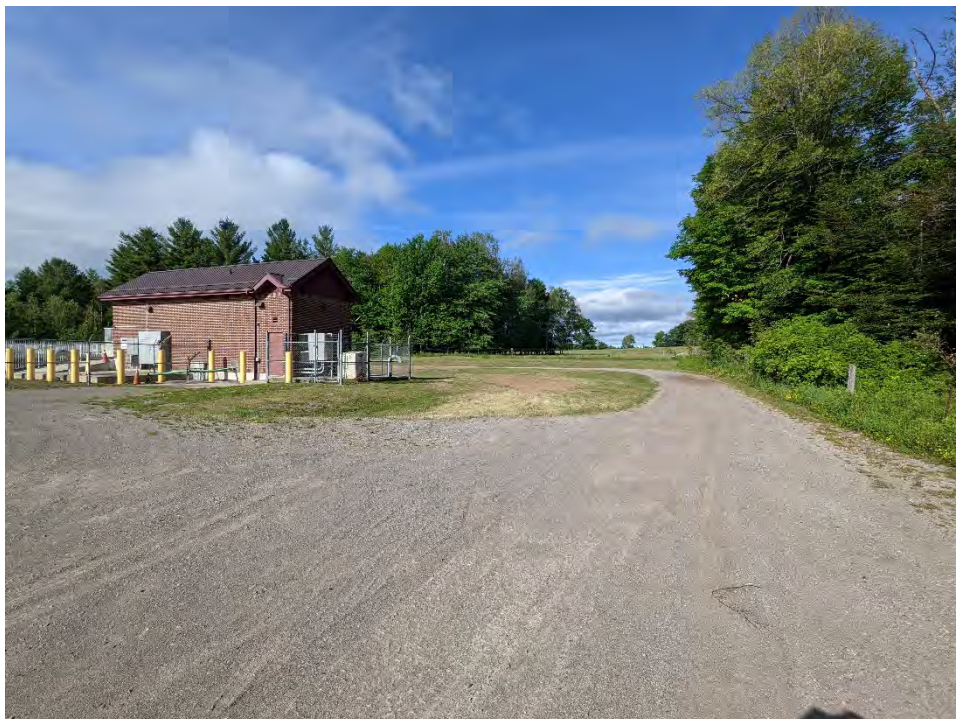
Image 2: Disturbed. Gravel road network and above ground facilities, looking southwest
