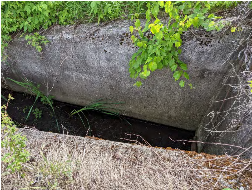
Image 10: Sewer utilities, looking down
