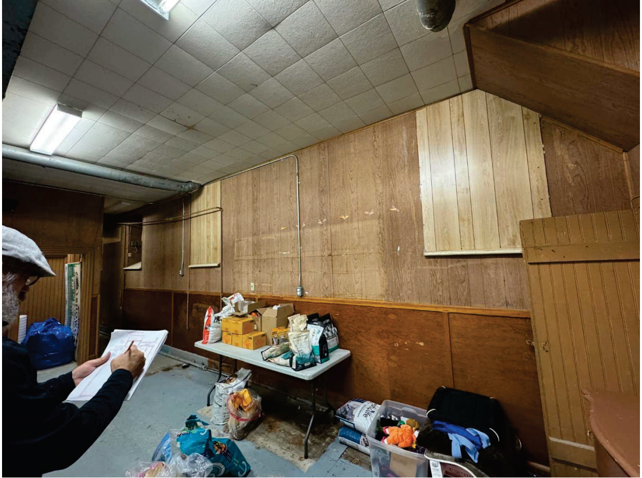
Photo #49 Basement east wall, looking west.
