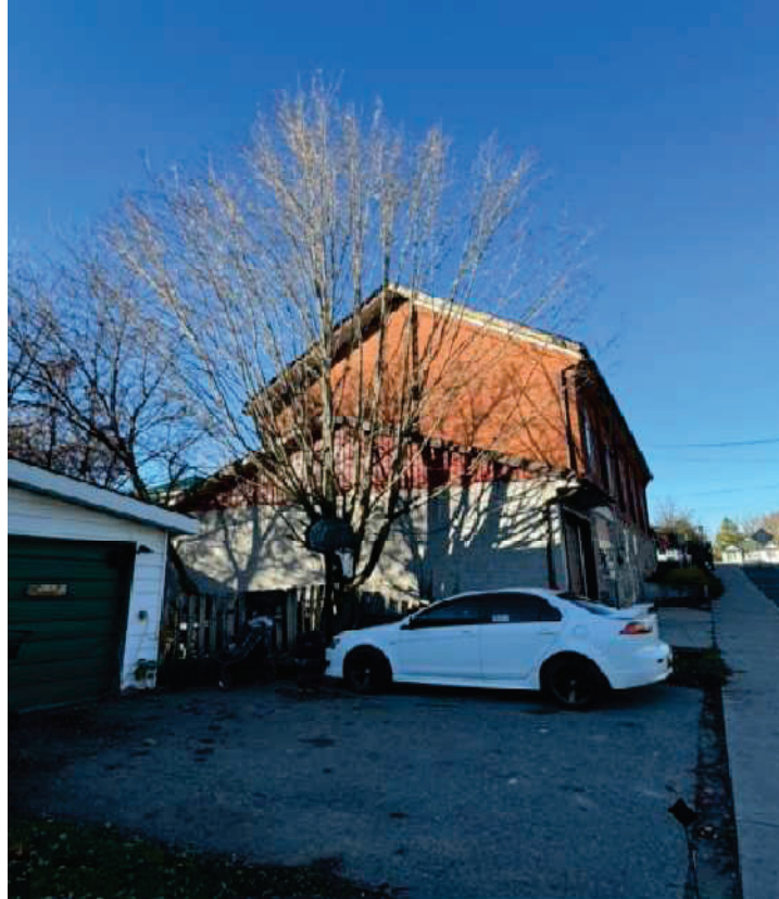
Photo #3 General View of the South Elevation
