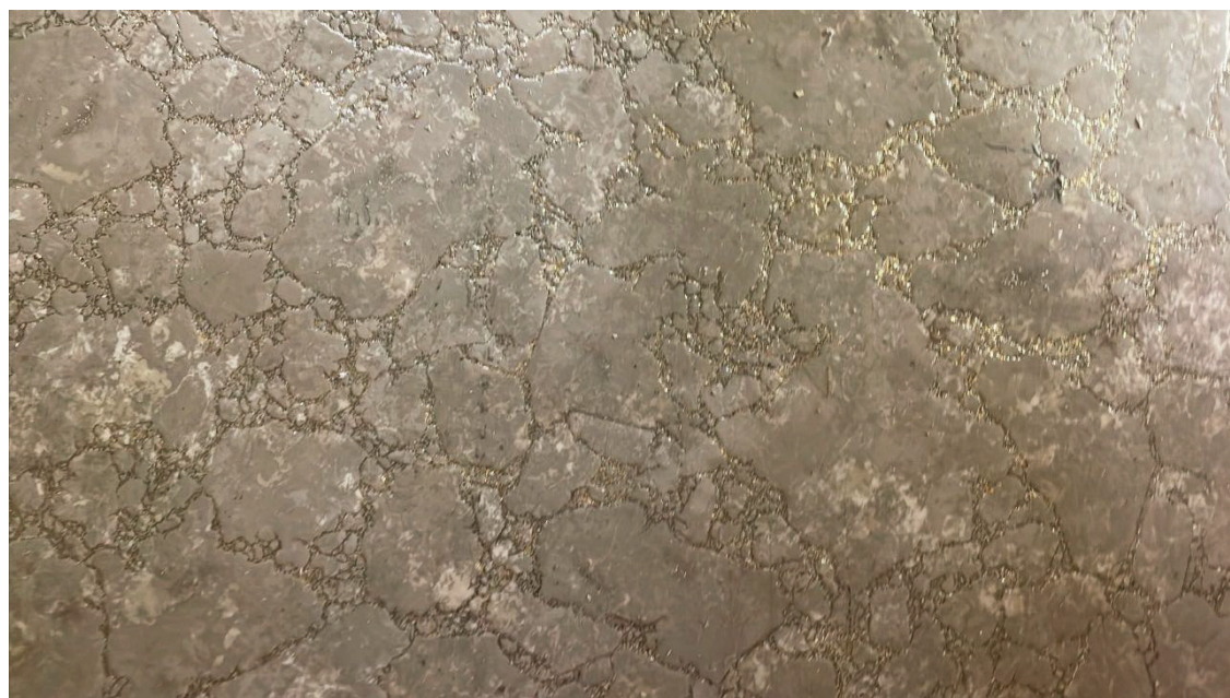
Figure 2: Asbestos-containing vinyl sheet flooring from Carpentry Shop
