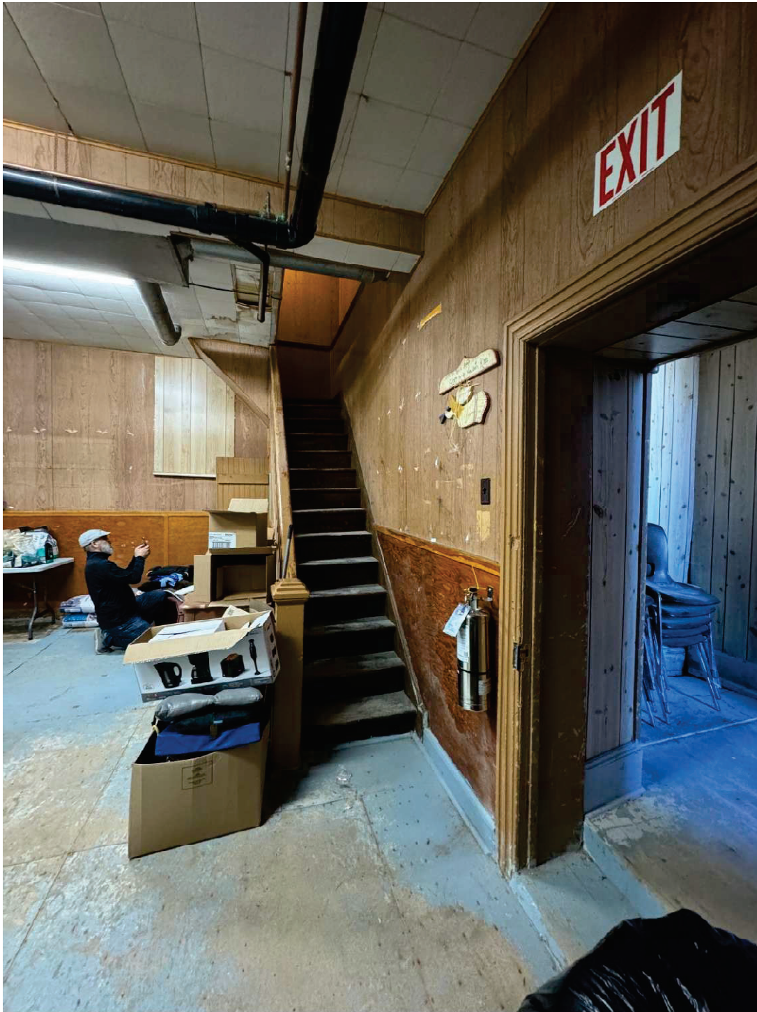
Photo #44 Basement North Exit/Access and North Stairs Leading to Ground Floor, Looking West
