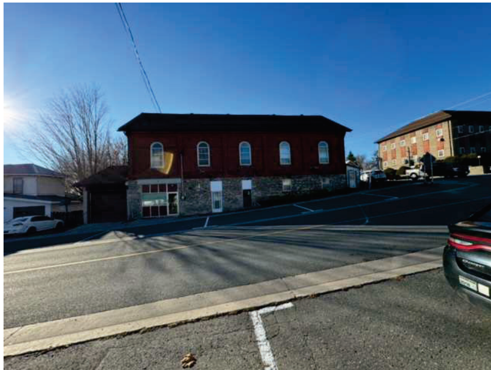
Photo #2 General View of the East Elevation
