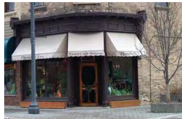
A corner flower store highlights windows and doors with permanent awnings. Note lower window boxes and simple yet effective signage on awnings.
