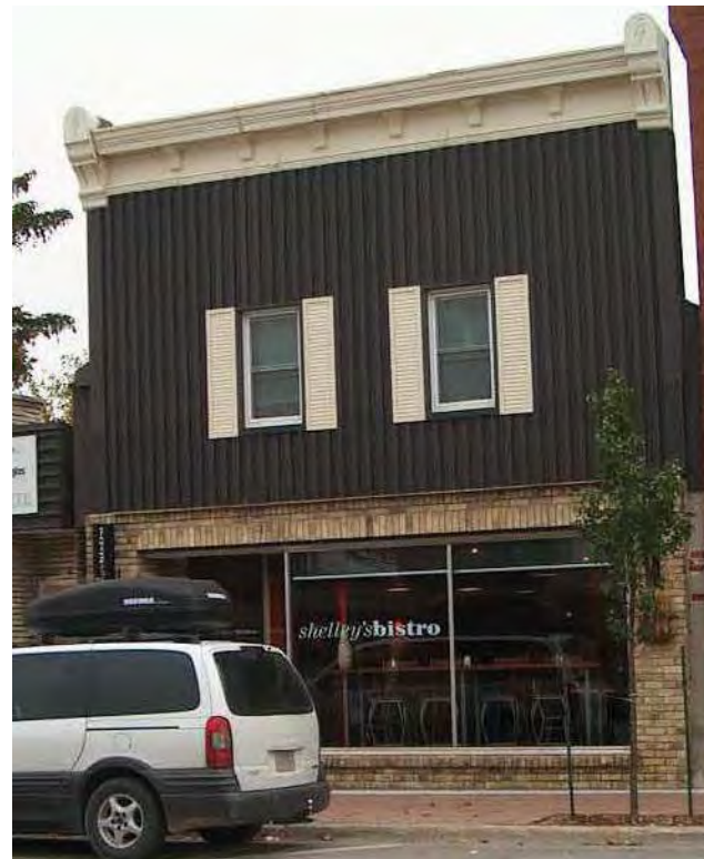
Contrasting vinyl shutters on upper windows. Note: Combination of vinyl siding with historic brick.
