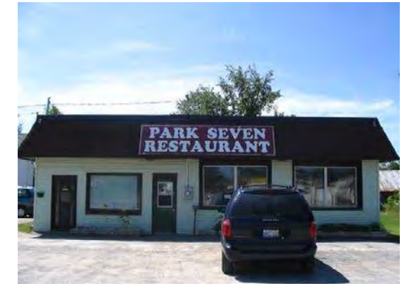
Park Seven Restaurant Havelock Facade Improvements
