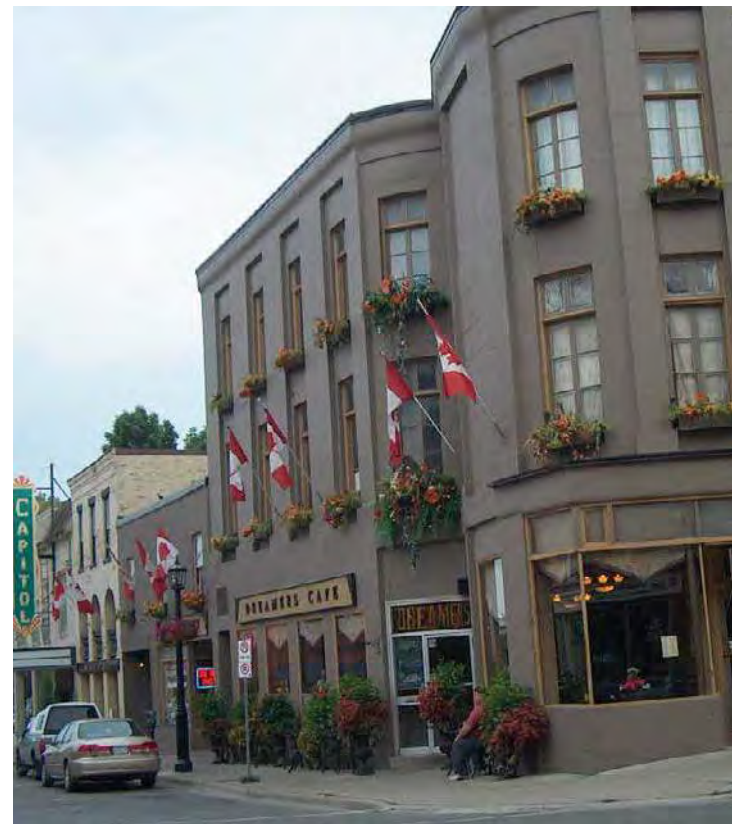
Co-ordinated window boxes on upper levels and urns along street
