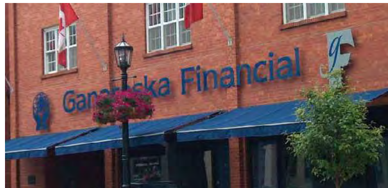
Painted metal letters and logos mounted directly onto building
