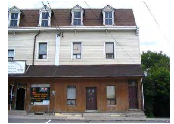
Cottage Country Books Havelock Facade Improvements
