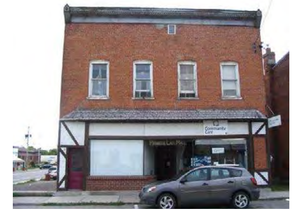
Community Care Havelock Facade Improvements
