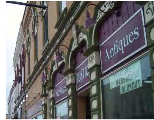
Traditional gooseneck lighting painted to match building colour scheme.
